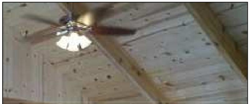
The Phase 2 ceiling finish knotty pine boards are installed over the 3x12 rafters included in the Phase 1 log shell kit
