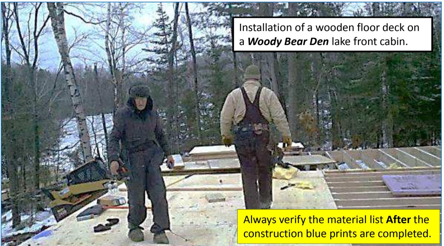
Installation of a wooden floor deck on a **Woody Bear Den** lake front cabin.
